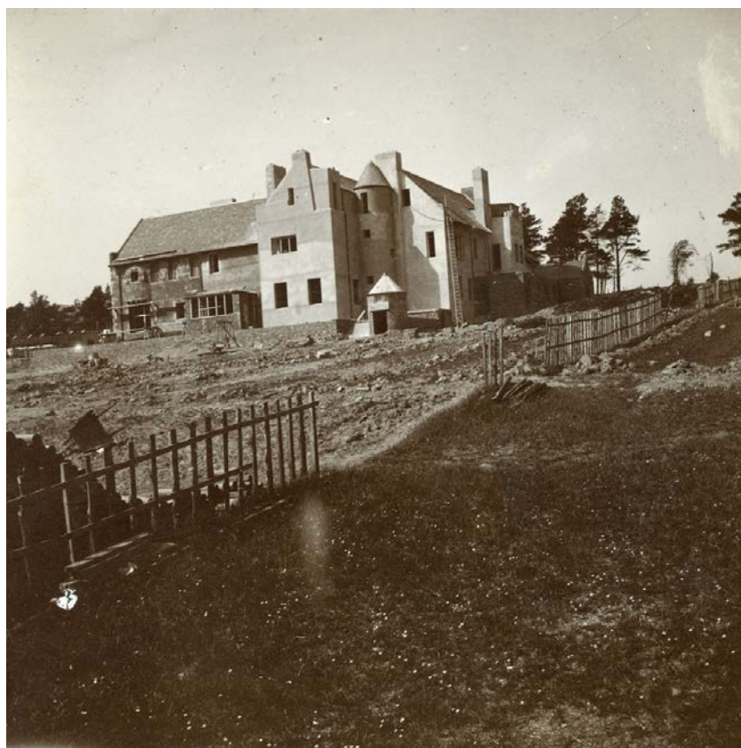
Photograph of The Hill House under construction (Summer 1903) with the roughcasting underway and the roofs already slated with the exception of the conical roof to the garden store © NTS
