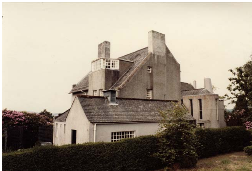
The north single storey range and northeast gable prior to repairs being undertaken in the mid-1980s: the full extent of repairs to the roughcast to the skewes and chimneyheads can be seen clearly © NTS
