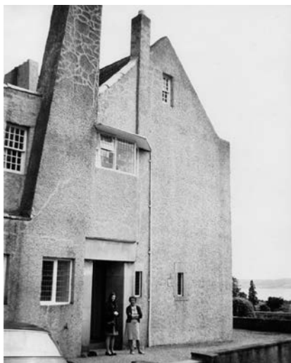
Above: the west elevation photographed in 1969, showing the extent of the pointing up of the cracks in the failed roughcast finishes; lead can be seen dressed over the skewers between the two chimneyheads and at the parapet at the flat roof, left (courtesy of Kenneth Lawson)
