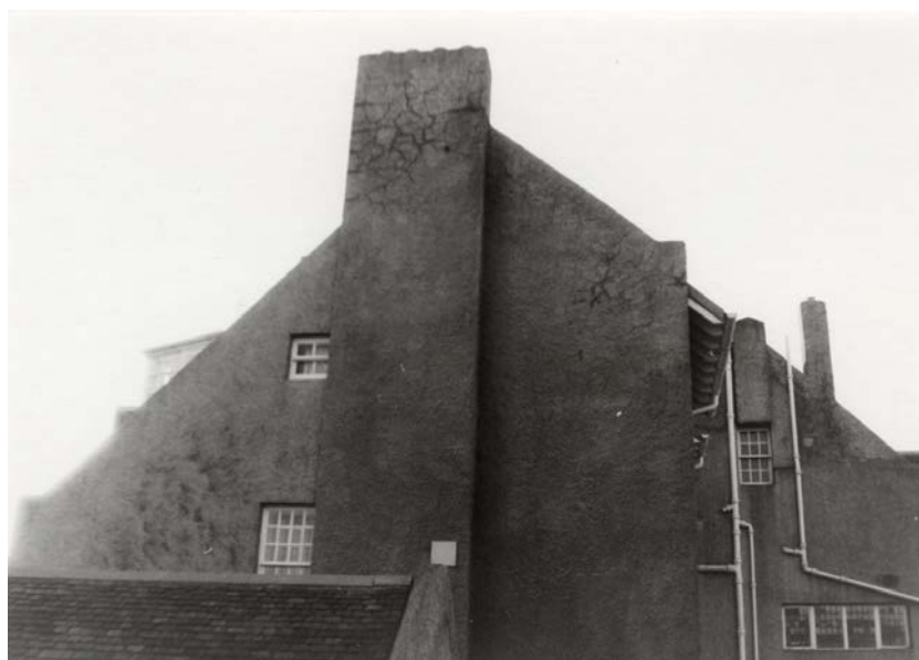
Right: photograph of the northeast gable taken before the house was handed over to the RIAS, but before the chimneyhead was removed at the middle gable (to the right of the picture), showing extensive problems with the roughcast of the gable © NTS
