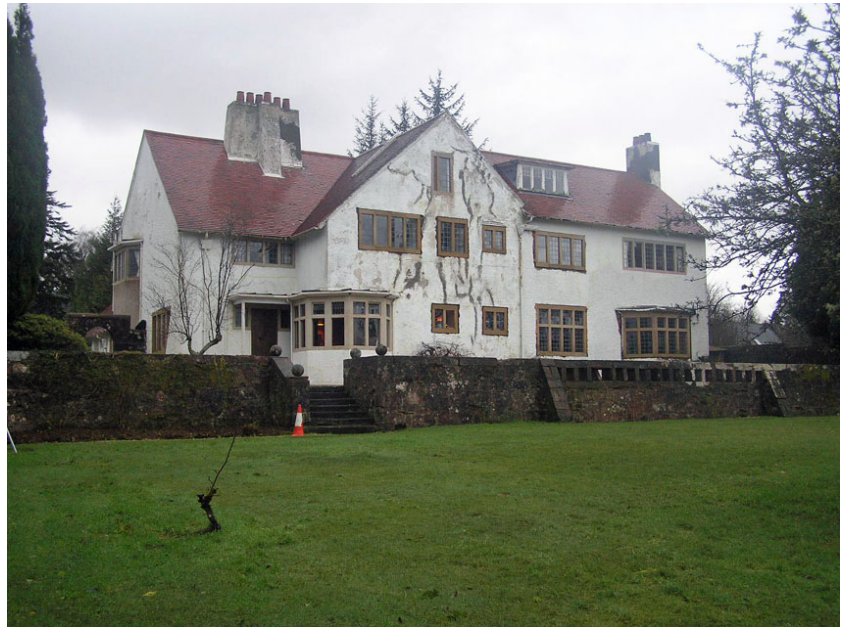
The White House in 2011, with repairs to the roughcast and replacement of stonework at windows underway: with the loss of the double height hall the fenestration has changed and the central chimneyhead has been removed. (Photo: author)
