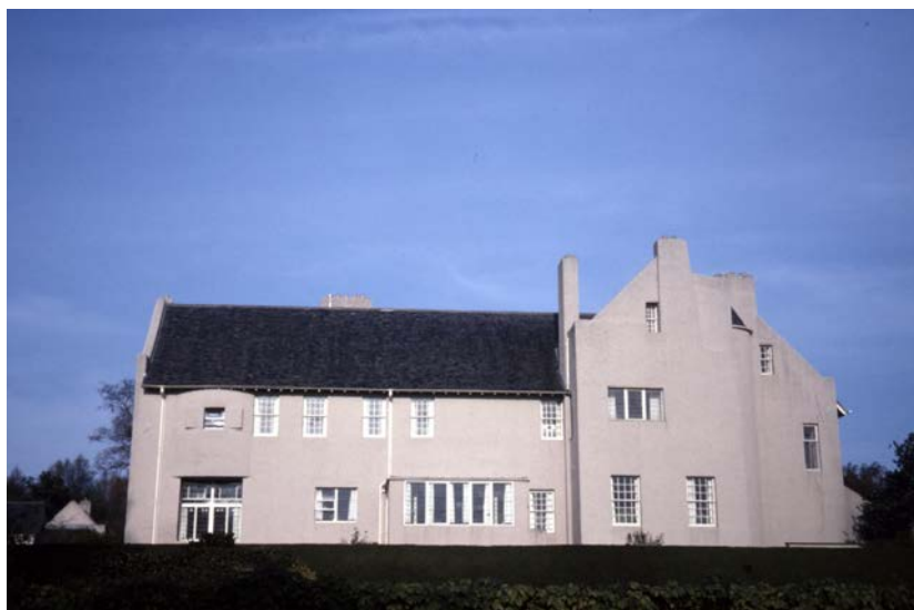
South (garden) elevation after the repair programme had been completed under Page & Park Architects © NTS
