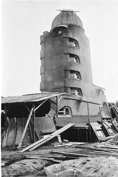
Top: the Einsteinturm shortly after completion in 1924 suggests a self-coloured Portland cement finish to the external surfaces (from Bennett, Plate LXIII 204 )
