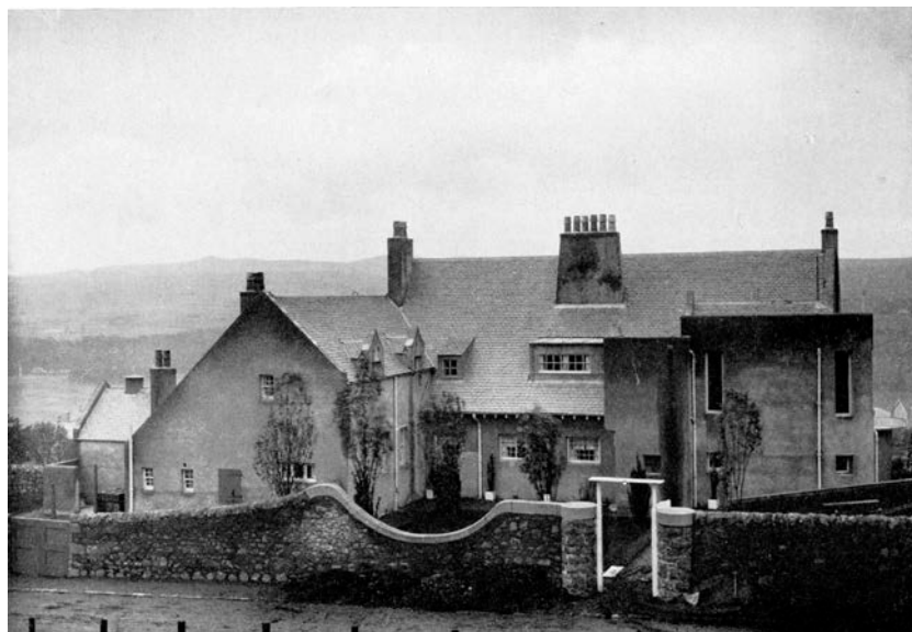
Windyhill , seen on a dull day from above the public road to the east of the site: within a few years after completion there are problems with the overflow from the secret gutter at the entrance tower, and the chimneyheads are harbouring dampness despite the inclusion of orthodox stone copes (from Howarth, Plate 34A)
