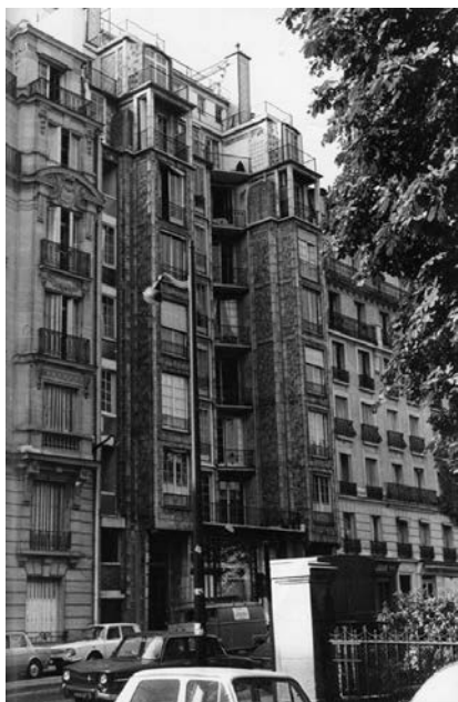
Auguste Perret's exposed reinforced concrete framed façade at 25 bis Rue Franklin, Paris (1903) (Photo: author)
