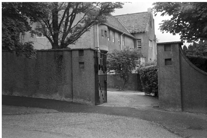
Right: photograph by David Walker (1959) shows the extent of crazing clearly in the area of the projecting window bay of the west elevation; where the beam to the curved bay on the south elevation has been replaced; and the reworking of the roof at the south gable to eliminate the chimneyhead and parapet in this area, where disturbed areas of roughcast can be discerned © Crown Copyright RCAHMS: licensor www.rcahms.gov.org
