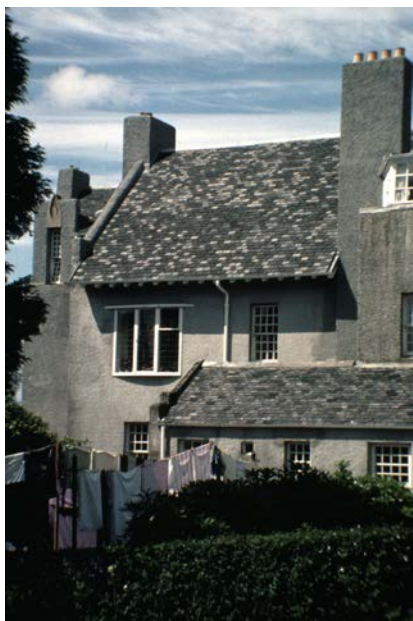
Partial view of the east elevation shows where recent repairs have been undertaken to the roughcast; new fenestration has been introduced to the single storey wing and the speckled appearance of the roof reveals that this has been reslated with salvaged material with the slate having the lighter colour originating from a different quarry © NTS
