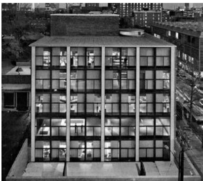
Top: Yale University Art Gallery (Louis Kahn, 1952-53) before refurbishment
